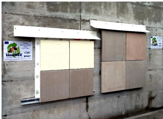
Figure 1 – Installation test of ETICS-like and ventilated façade panels on a free-standing wall
